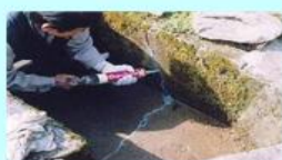
ひび割れ補修
